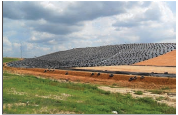
Temporary Landfill Cover
