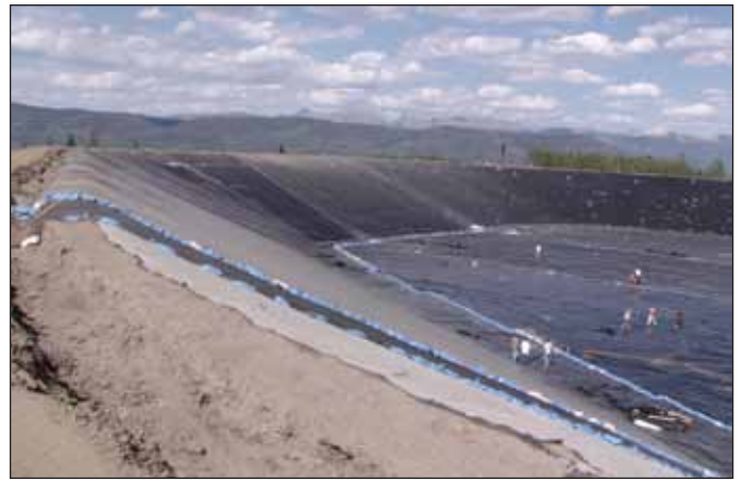
Containment Pond Liner
